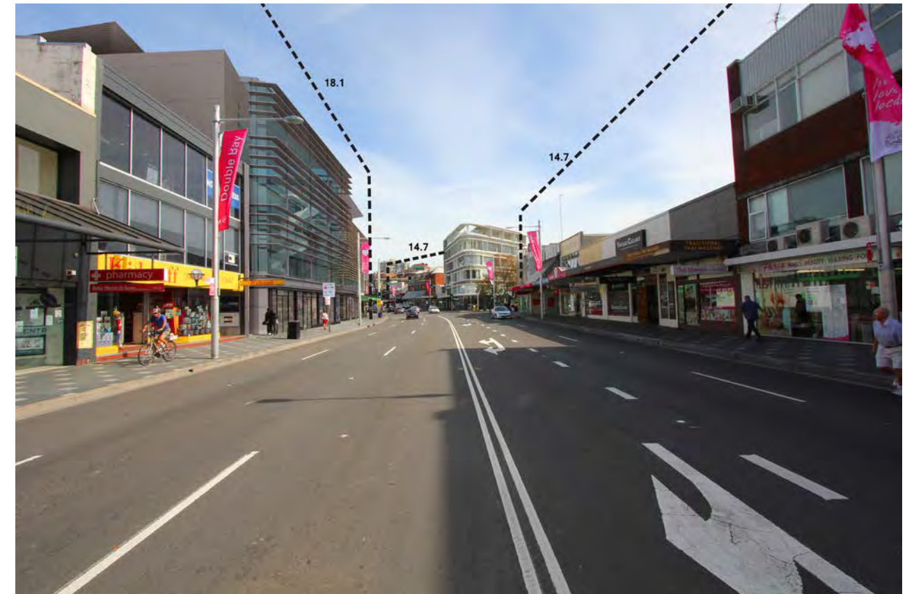
FIGURE 1: NEW SOUTH HEAD ROAD
